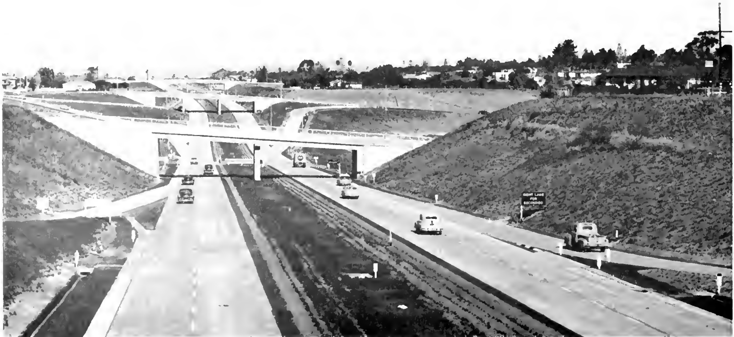
Looking north along a portion of the Oceanside Freeway, showing some of the grade separations and interchange ramps which have contributed to a sharp reduction in accidents since opening of the freeway on November 16, 1953
